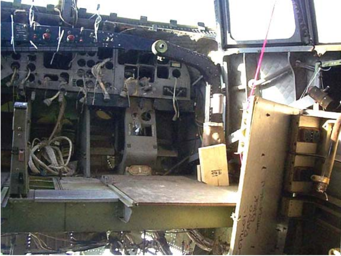
The deplorable condition of the cockpit control panel is evident in this image taken before work was begun. All instruments are missing and at the bottom we can see right through the hole in the nose section where work on the wheel well had stopped - leaving the interior of the aircraft wide open to the elements and fauna of South Carolina for years. Photo via www.buffalo461.ca
